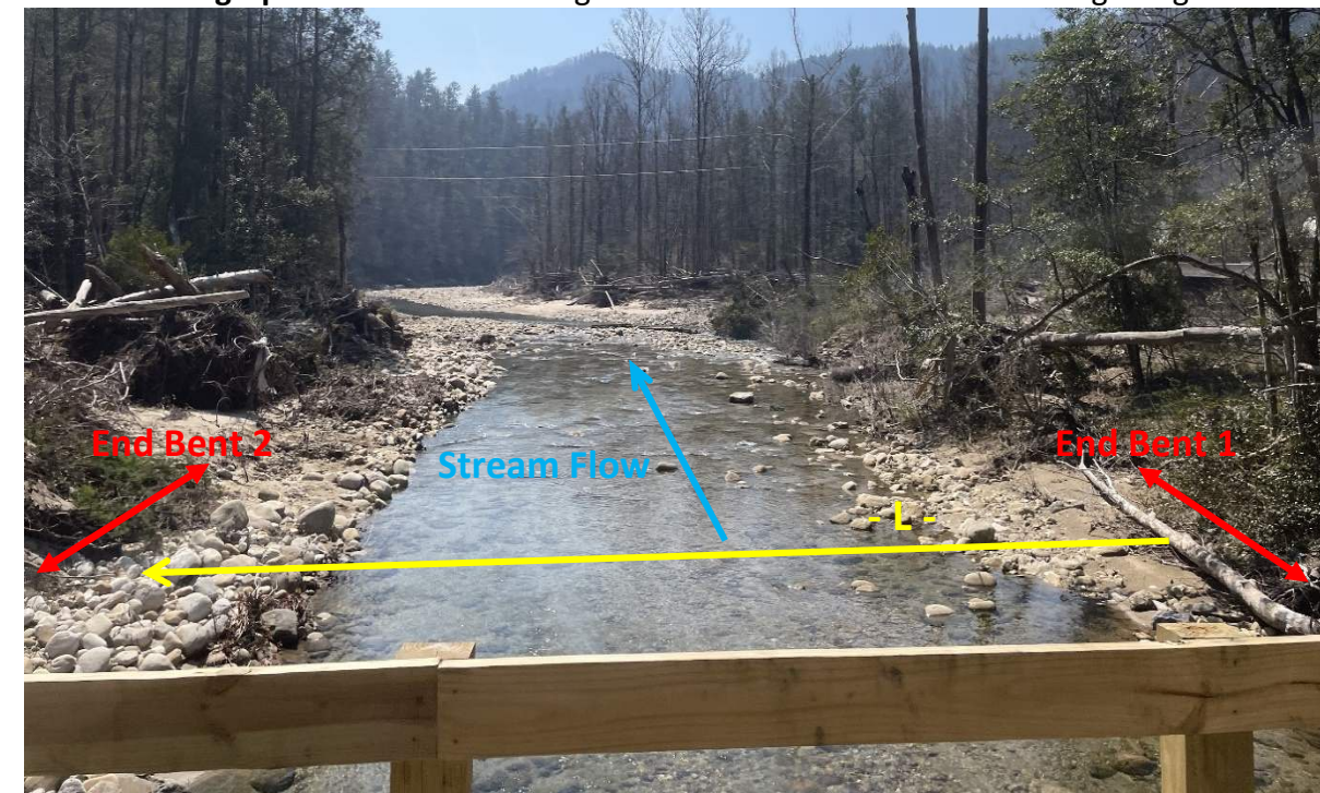
Photograph No. 4: Looking south downstream at the existing bridge
