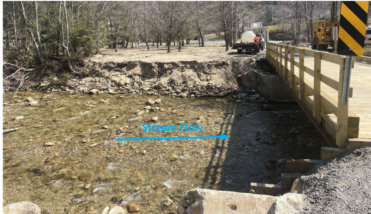
Photograph No. 1: Looking east at the beginning of the existing bridge
